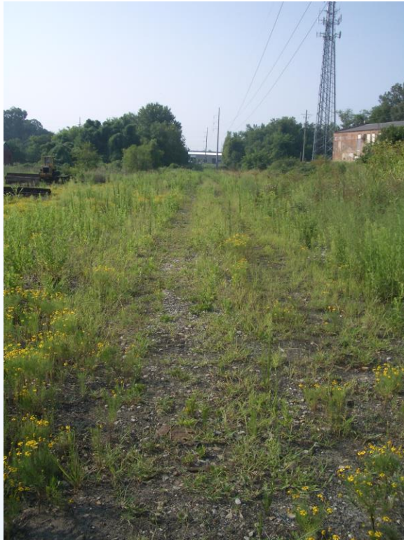
Decommissioned Rail Line
