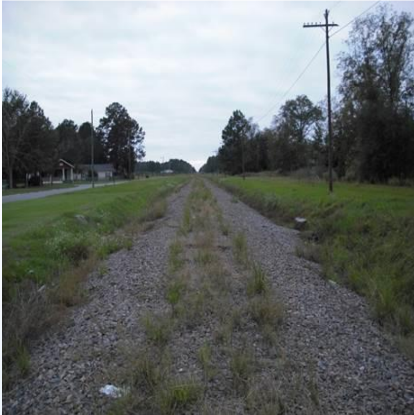
Decommissioned Rail Line
